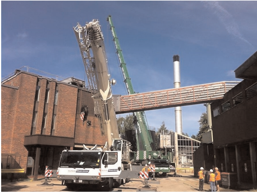
Figure 5. Removal of one of the tanks, 2016. Photo by the author.
