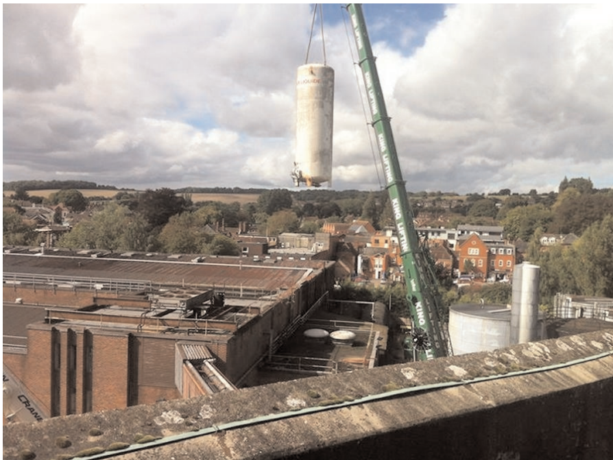
Figure 6. Removal of one of the tanks, 2016. Photo by the author.
